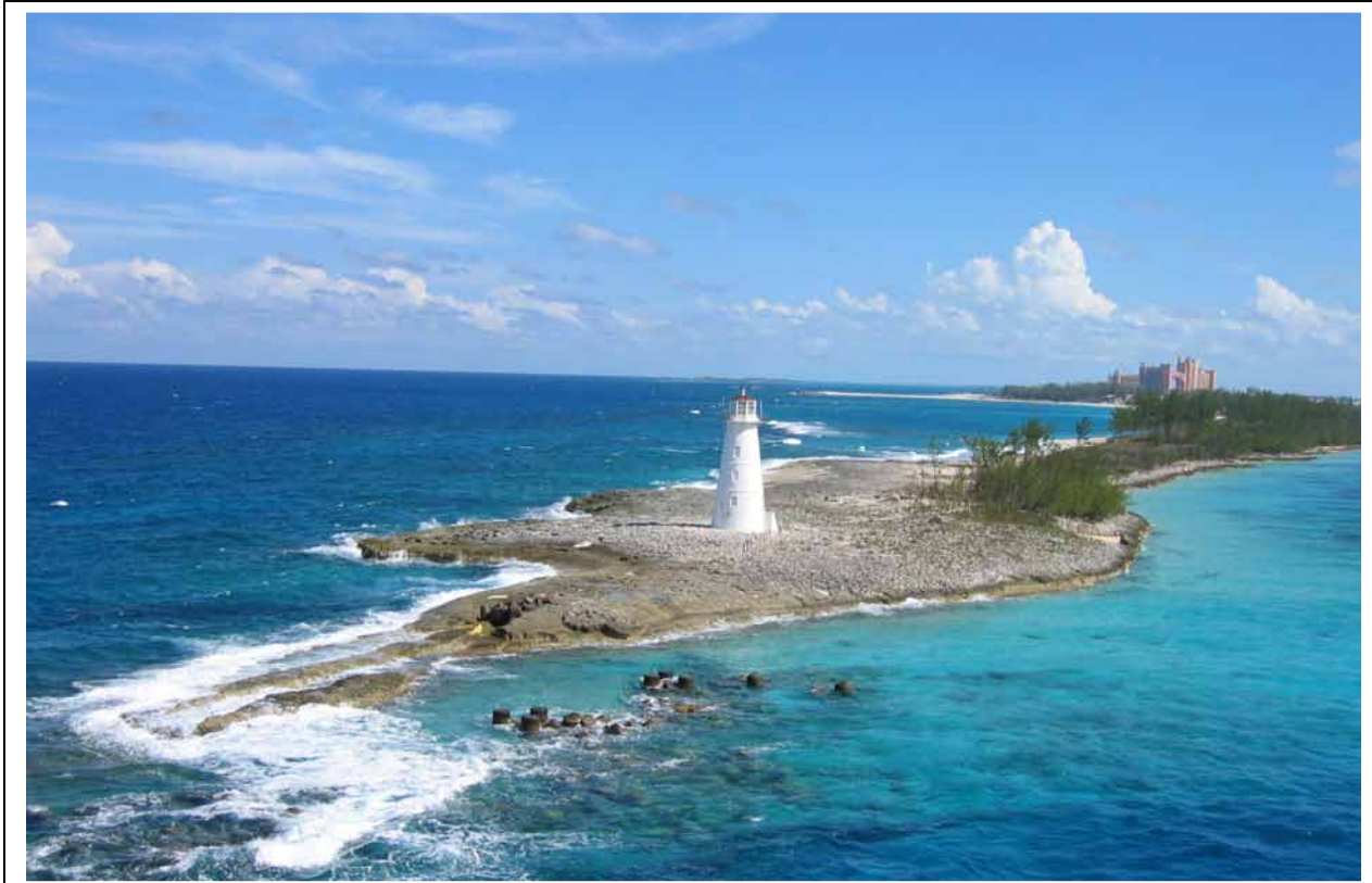
Photo 2: East breakwater looking east from damaged section
