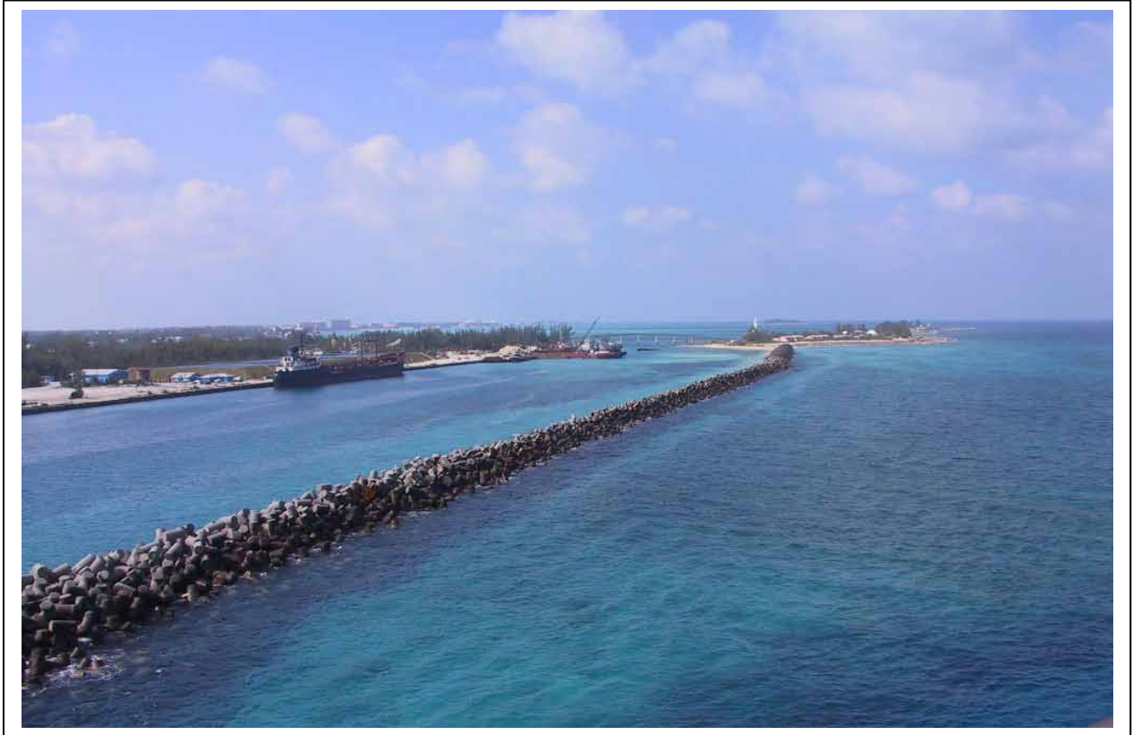
Photo 1: West breakwater looking west
