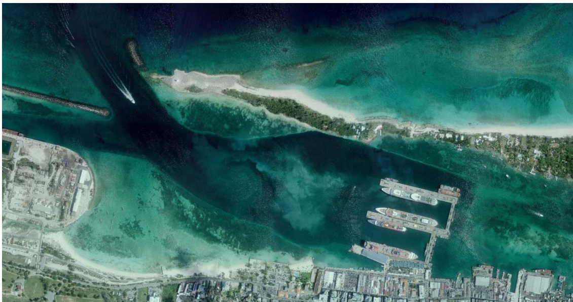
Figure 1.1 Aerial Image of Nassau Harbour Main Navigation Channel
