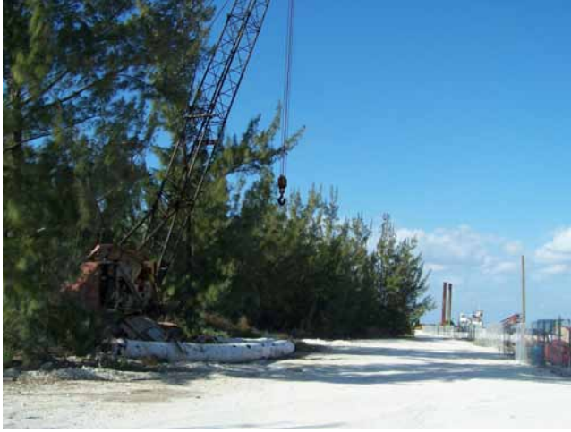
Item 10. Abandoned damaged concrete
